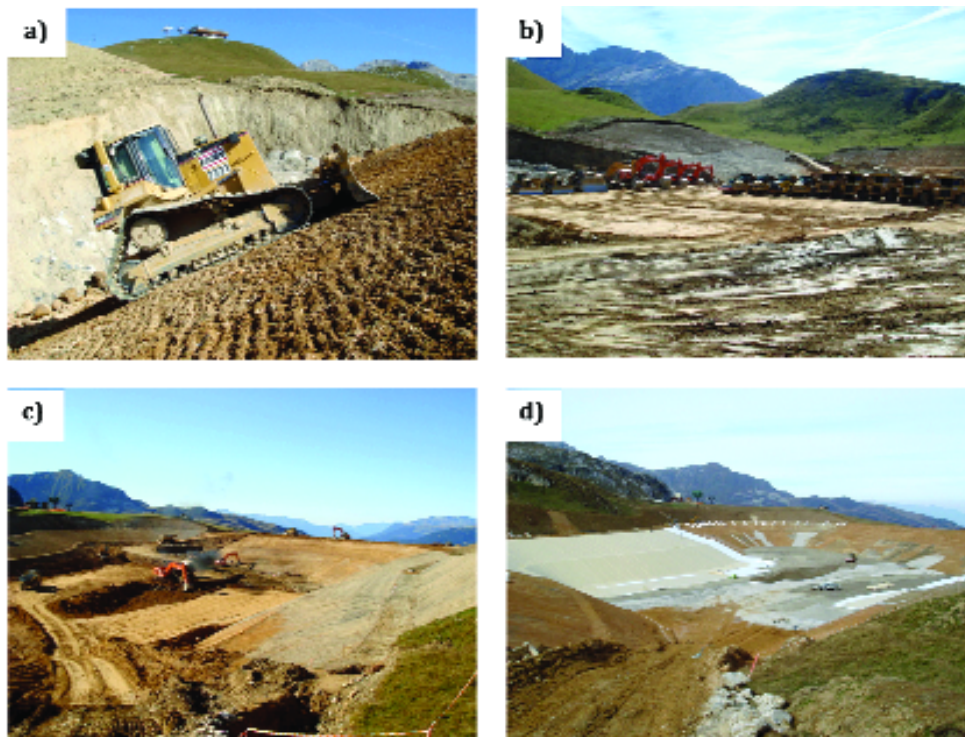
Figure 6 Construction of the new Ariondaz reservoir (125 000 m 3 in size at 2500 m a.s.l) to store water for artificial snow production for ski runs in Courchevel, French Alps in 2007.
